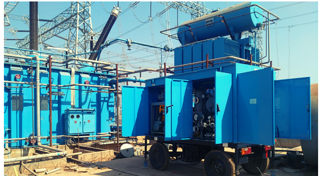
Ultra High Vacuum Transformer Oil Filtration M/c (JHVR 10000X) at BHEL
